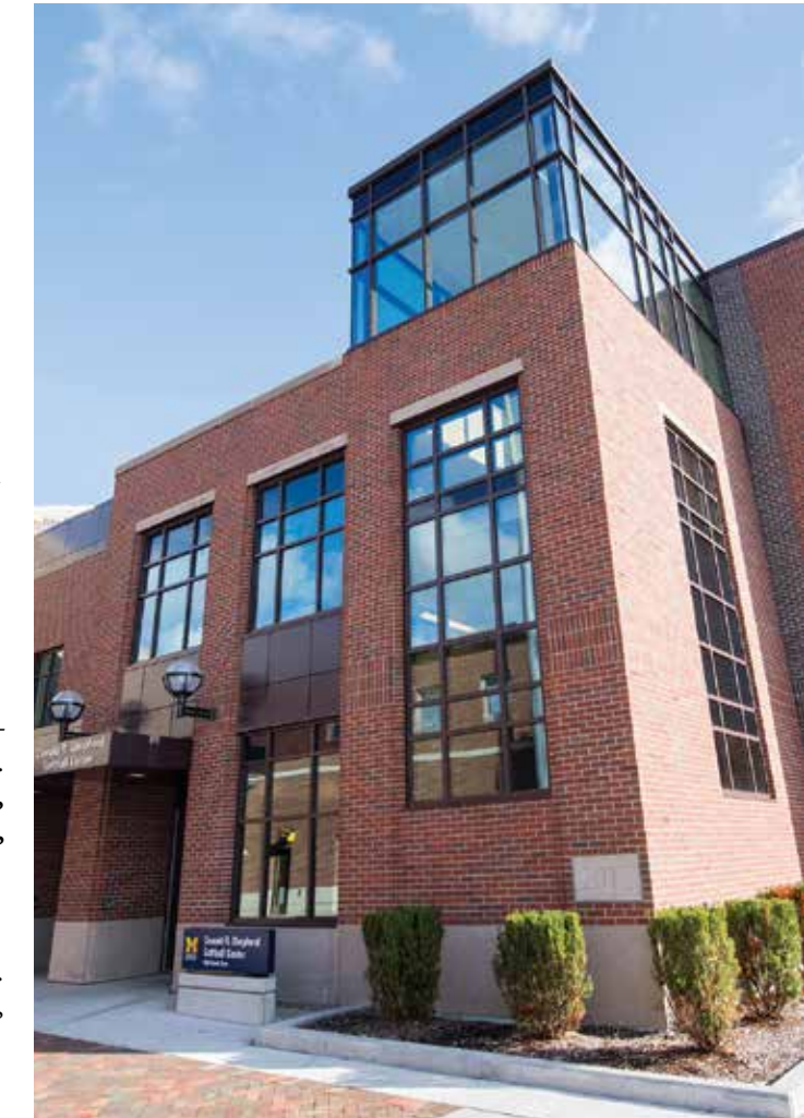
The Donald R. Shepherd Softball Center includes a museum, coaches' offices, improved training facilities, team meeting space, and a fitness room. The center is the latest addition to the Wilpon Complex, home to the U-M baseball and softball teams.
