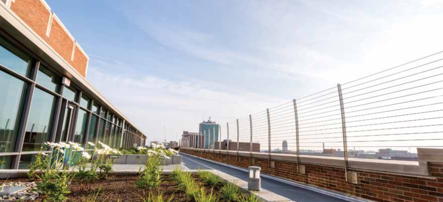
A view looking north from the rooftop running track at Munger Graduate Residences.
