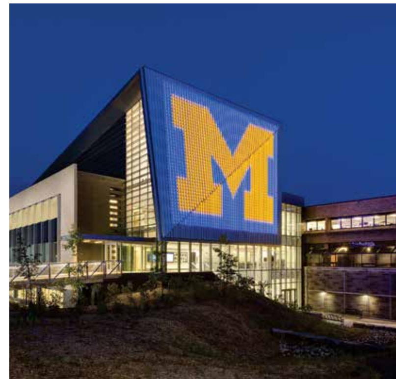
The Center of Excellence in Nano Mechanical Science and Engineering on U-M's North Campus
